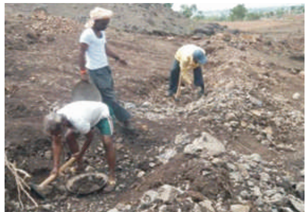
Figure 14. Constructed Contour trenching
