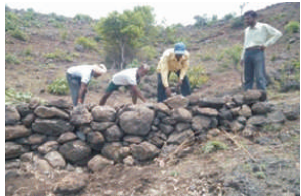
Figure 13. Constructed Gully Plugs
